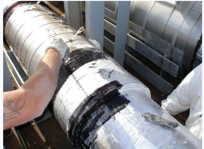
Cryogel Z tie-in to adjacent insulation material.
